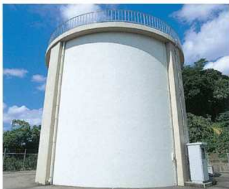
[緑ヶ丘配水池]
