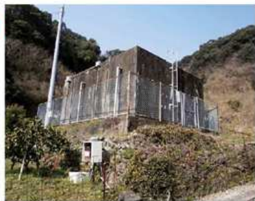
[平木場配水池]
