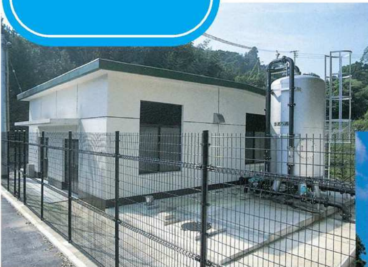
[東高田浄水場]
